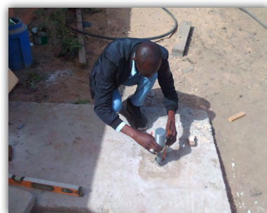
Figure 15: Fossetic technician installing a sensor to monitor septic tanks.
